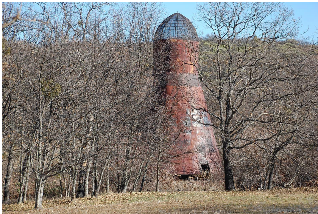
The last and only known “onsite” remnant of the Ayers Spur Community: the wigwam or teepee burner that was situated beside the planing mill. (2014 photo by T. Sayre)
