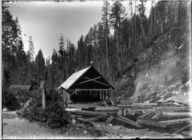
Logs being fed from the log pond to the steam-powered saw at the “Upper Mill.” (Photo courtesy of the Southern Oregon Historical Society; SOHS 2532)
